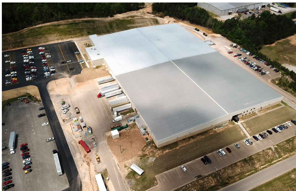
GE Appliances Monogram Refrigeration, LLC Plant in Selmer, TN.
